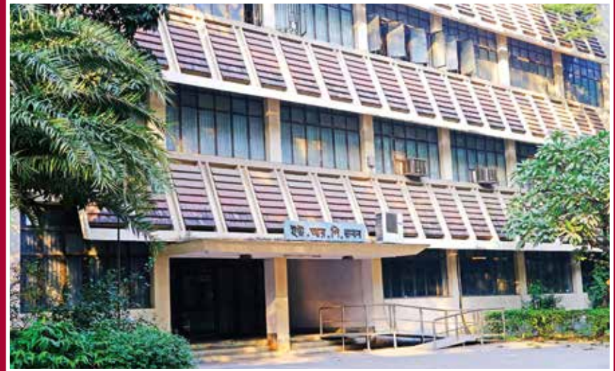
Urban and Regional Planning Building
