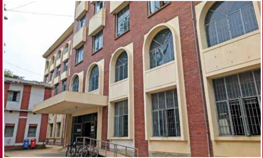
Controller of Examinations (CoE) Building
